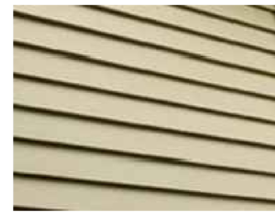
1 PROPOSED SIDING MATERIAL #1 PAINTED CEDAR LAP SIDING, COLOR REFERENCE PICTURED
